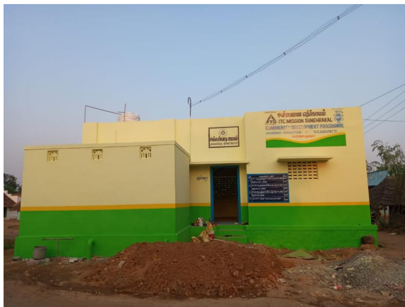
Photos of a renovated Anganwadi in Pudukottai District
