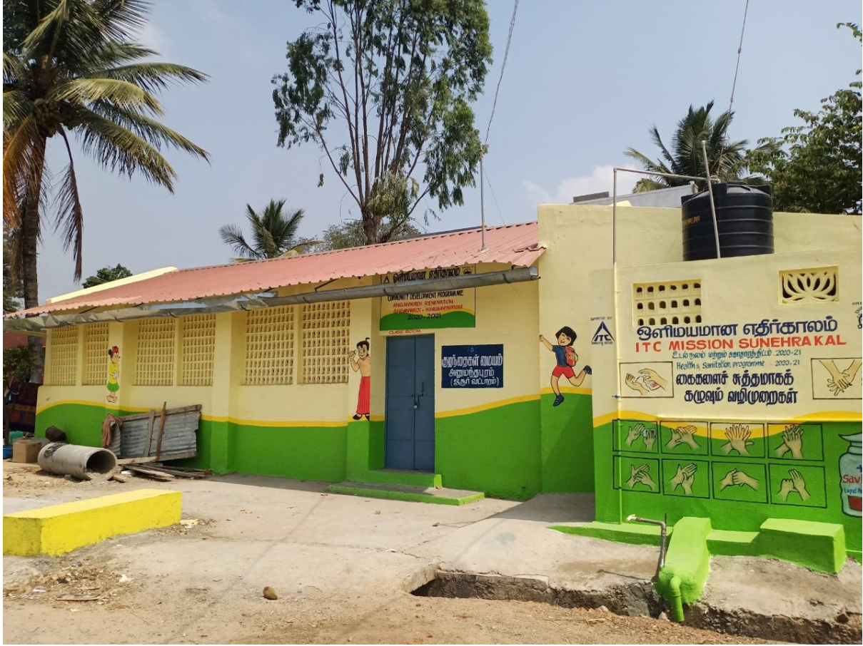
A renovated Anganwadi building at Hanumanthapuram village
