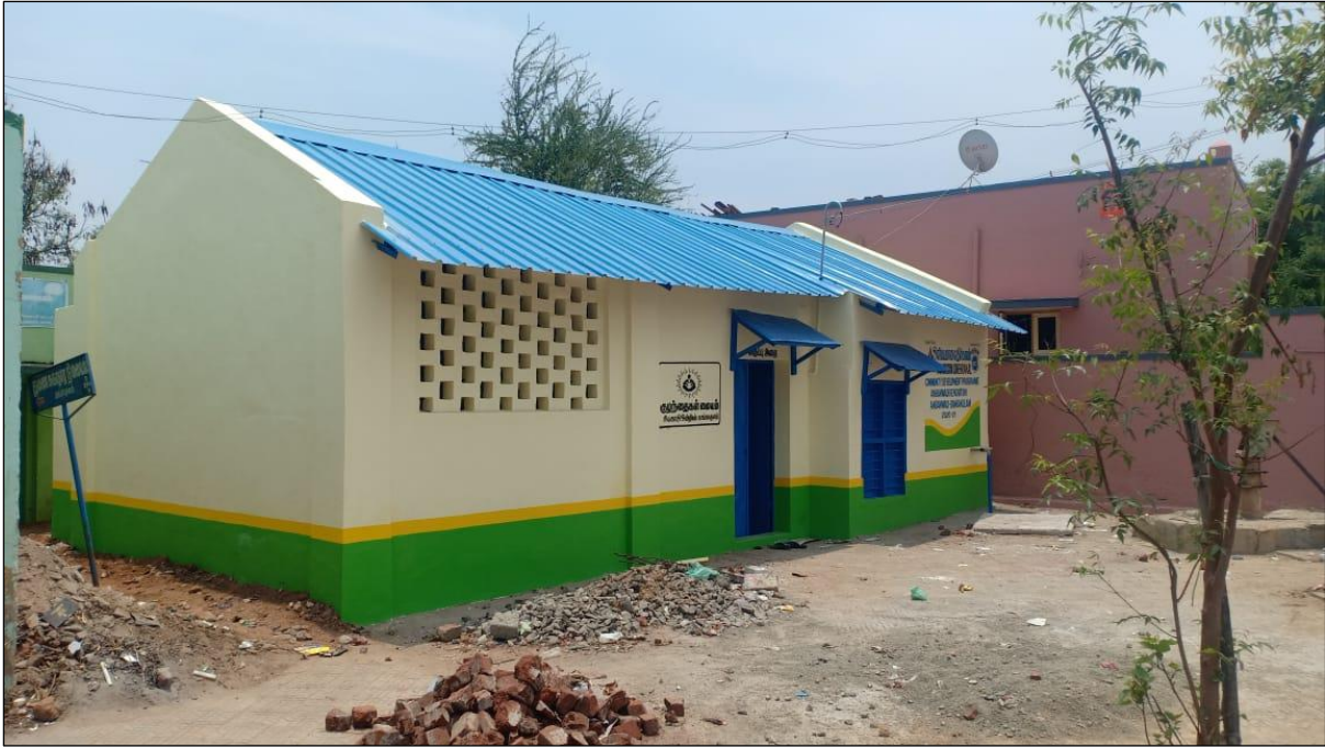
A newly renovated Anganwadi at Gangakulam Village, Sivakasi Block
